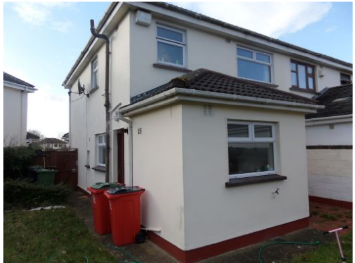
Rear extension added.
