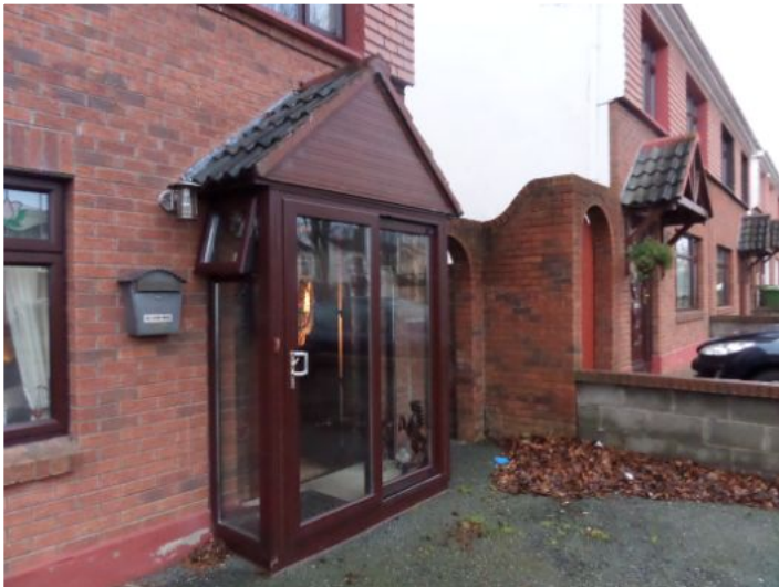
Front porch added.
