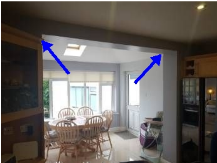
Wall removed between original house and extension.
