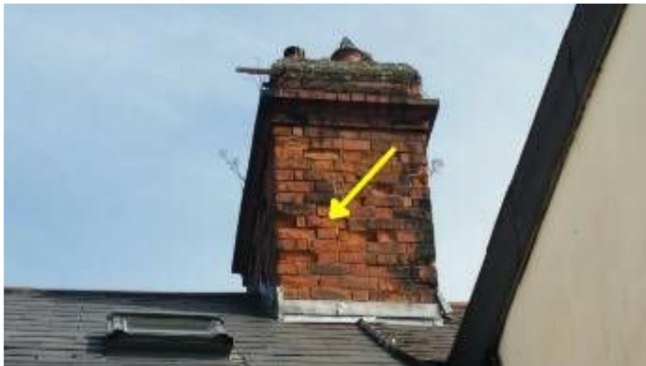
Spalling bricks.
