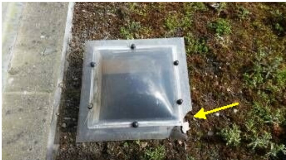
Damaged skylight.
