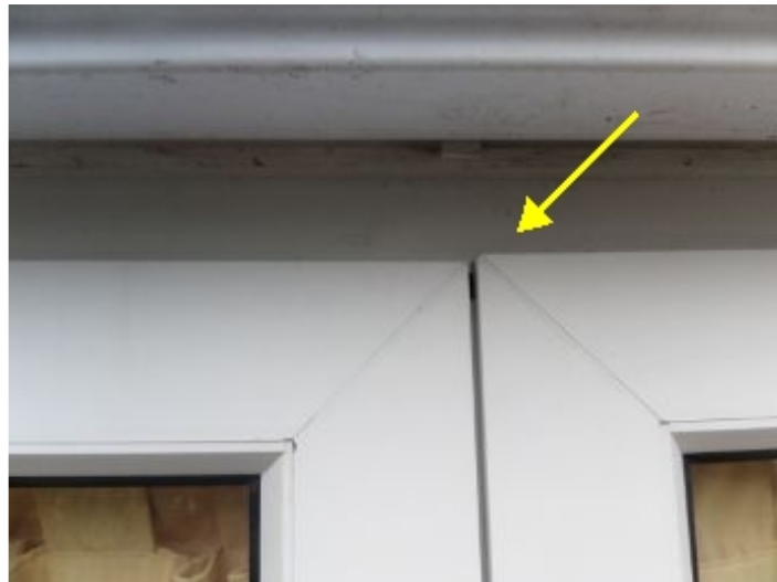
Back doors required re-alignment.
