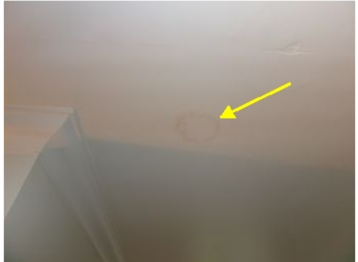
Moisture stains under bathroom.
