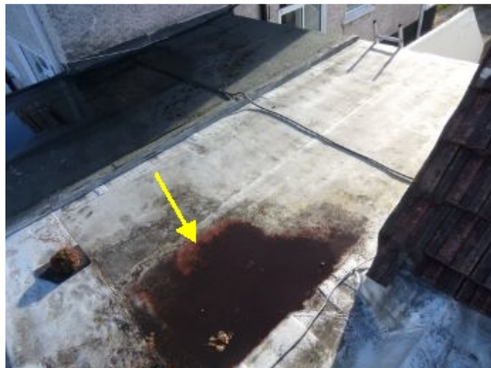
Water ponding on flat roof.
