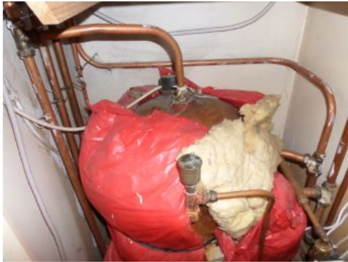
The hot water cylinder is lagged with a loose jacket.
