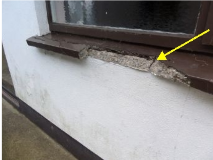
Window sill cracking to right side of house.
