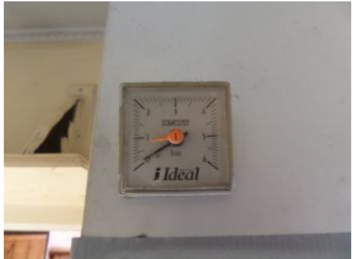
Low water pressure to heating system.
