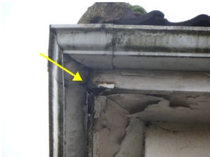
Rotting roof eaves.
