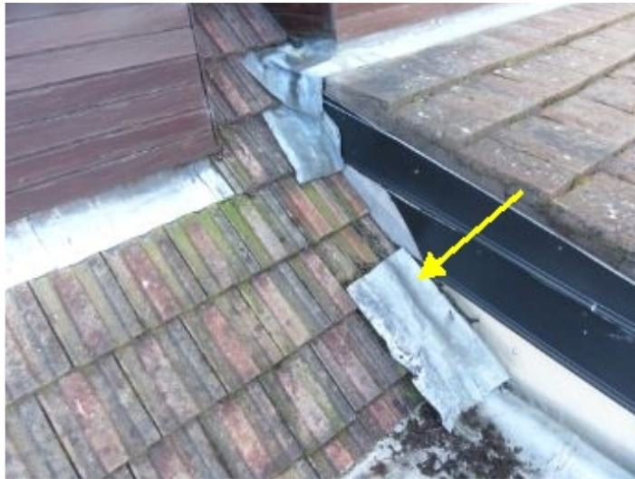
Flashing slipped / loose.
