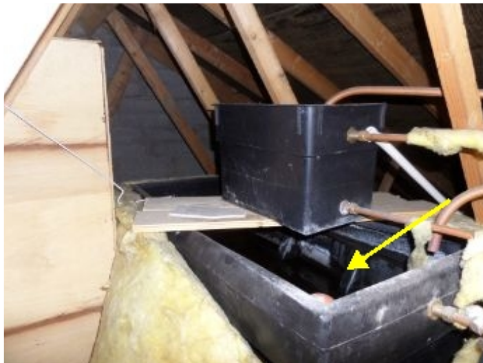
Cover required over water storage tank.
