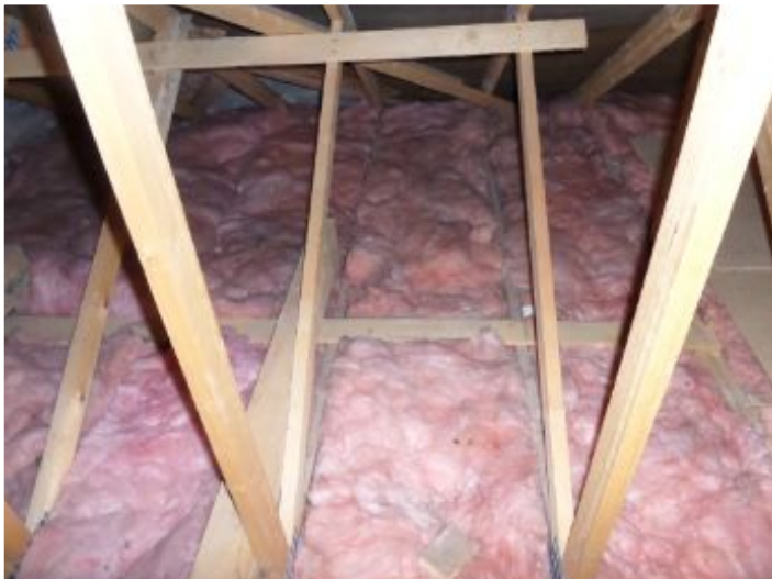
Approximately 100 -150mm of insulation on attic floors.
