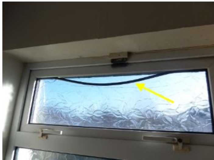
Window seal failing in double glazing to bathroom window.
