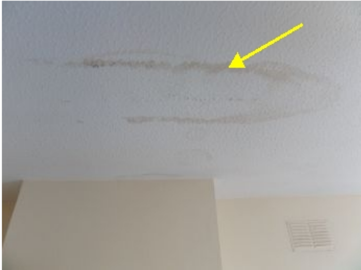
Moisture stain in ceiling at chimney.
