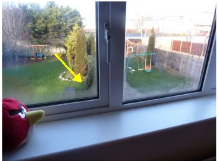
Window seals failing in double glazing at back of house, condensation noted.
