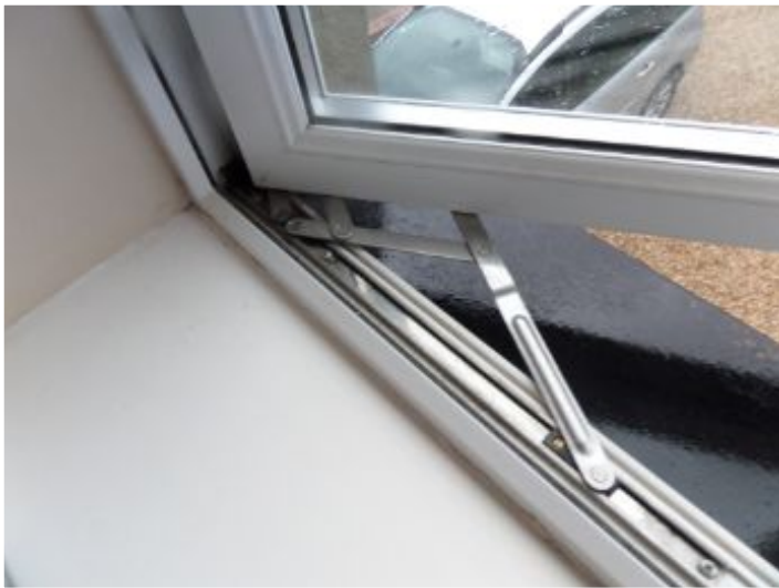
Window hinges require lubrication.
