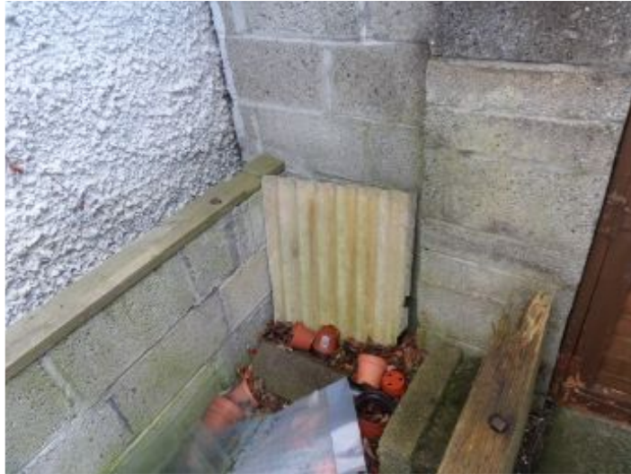
Asbestos panel noted in back garden.
