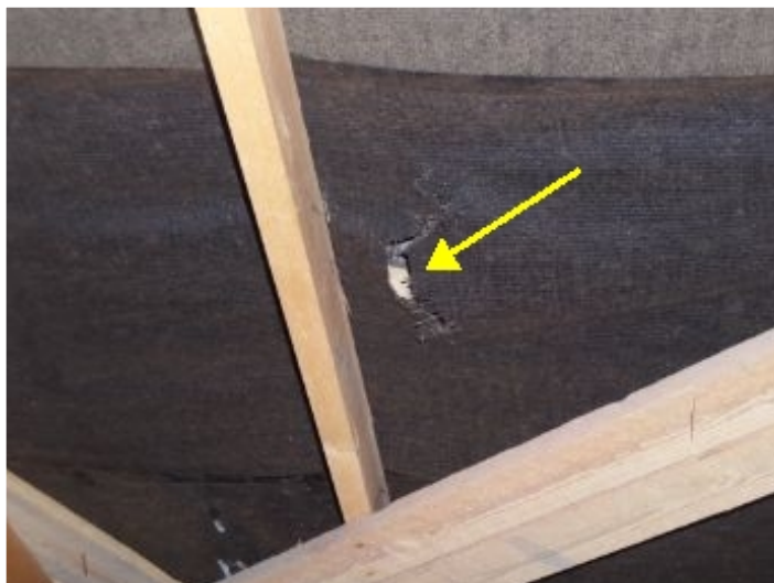
Hole / tear in roof felt.
