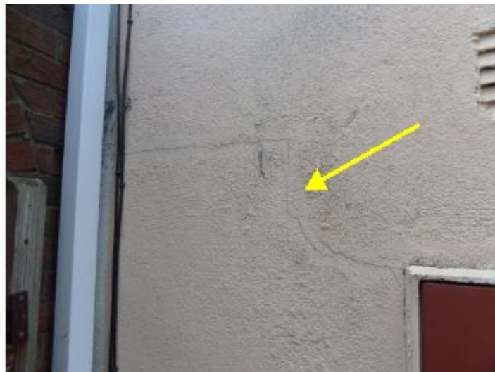
Thermal cracking in cement rendered walls.
