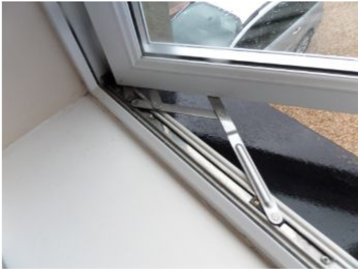
Window hinges require lubrication.
