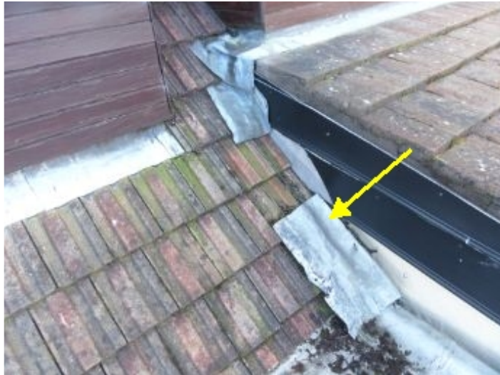
Flashing slipped / loose.
