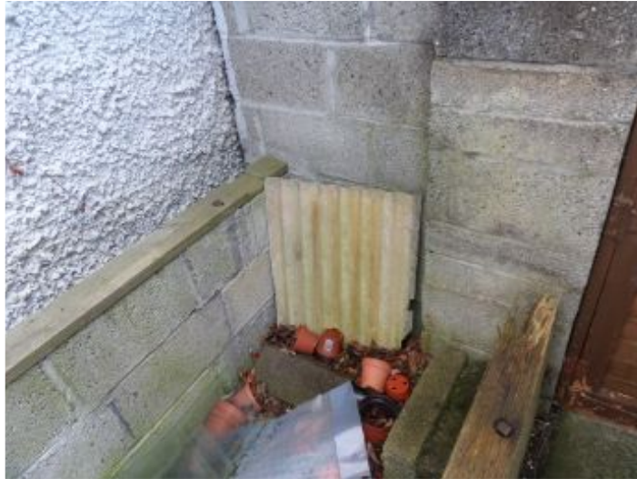
Asbestos panel noted in back garden.
