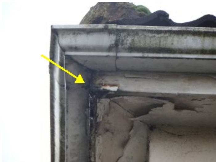
Rotting roof eaves.
