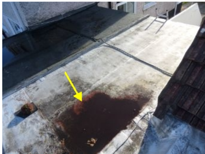
Water ponding on flat roof.
