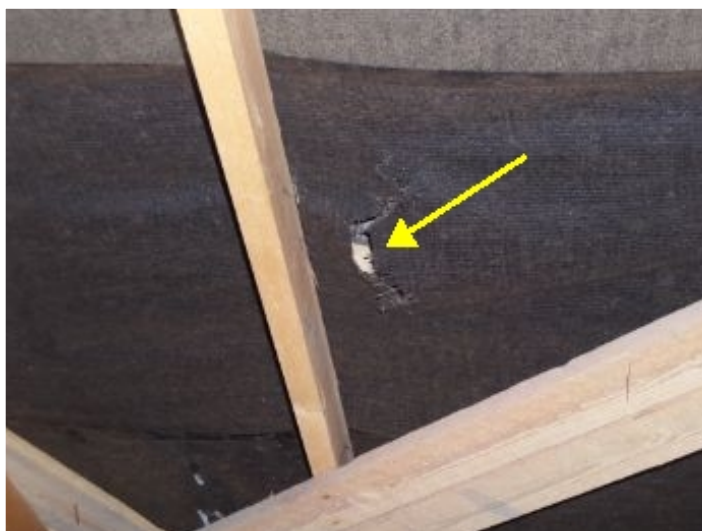
Hole / tear in roof felt.
