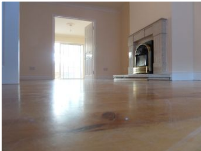
No unusual sloping / deflection was noted in the floors at the time of inspection.
