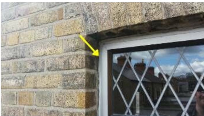
Re-seal around window frames to walls.
