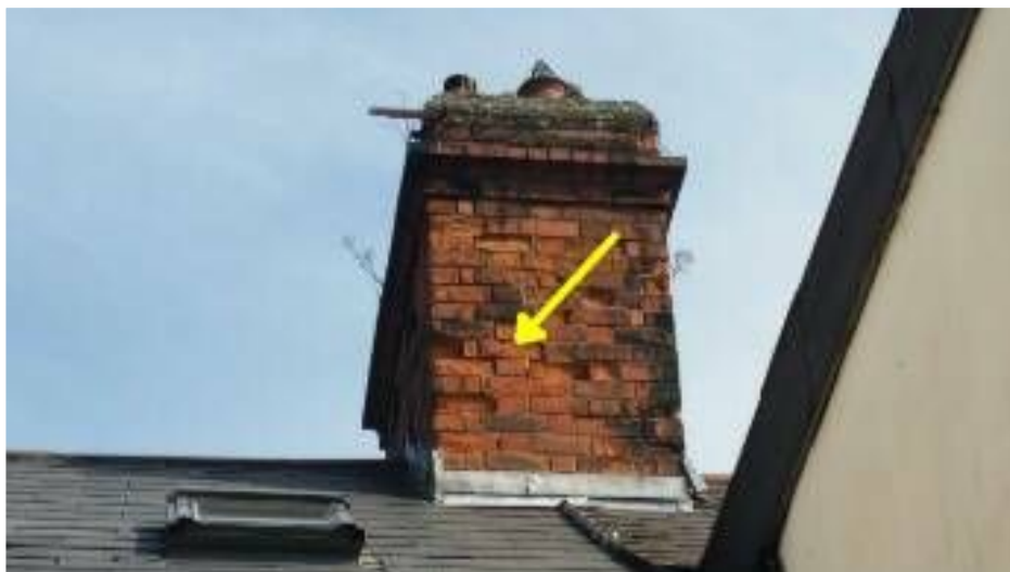
Spalling bricks.
