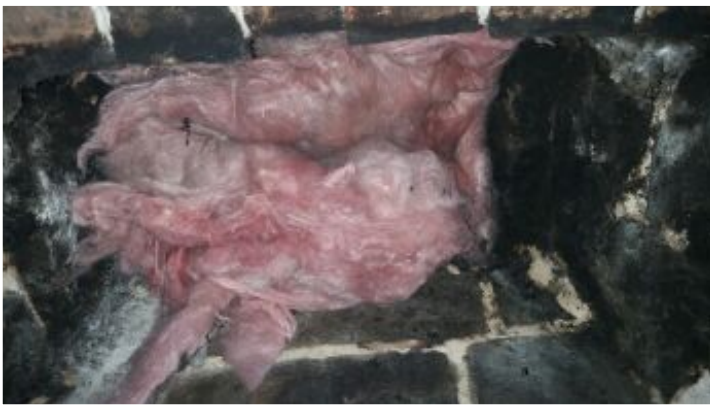
Fibreglas insulation stuffed up chimney. Clean out before use.
