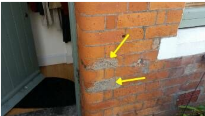
Bricks spalling.
