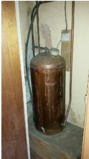
Aging copper cylinder.
