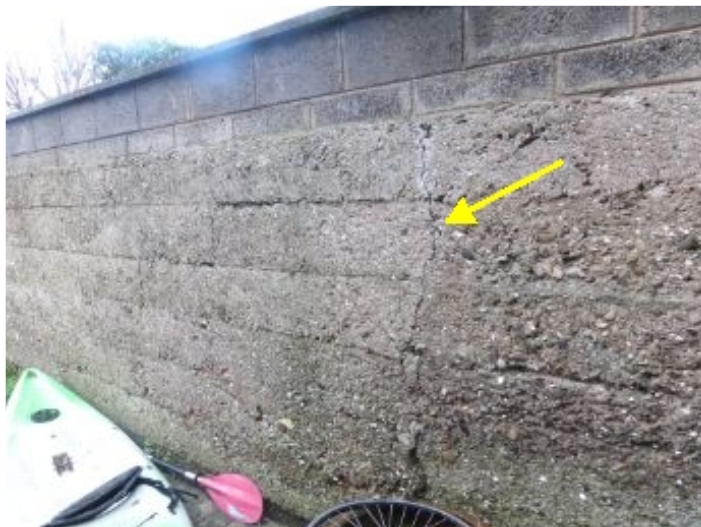
Crack in boundary wall.
