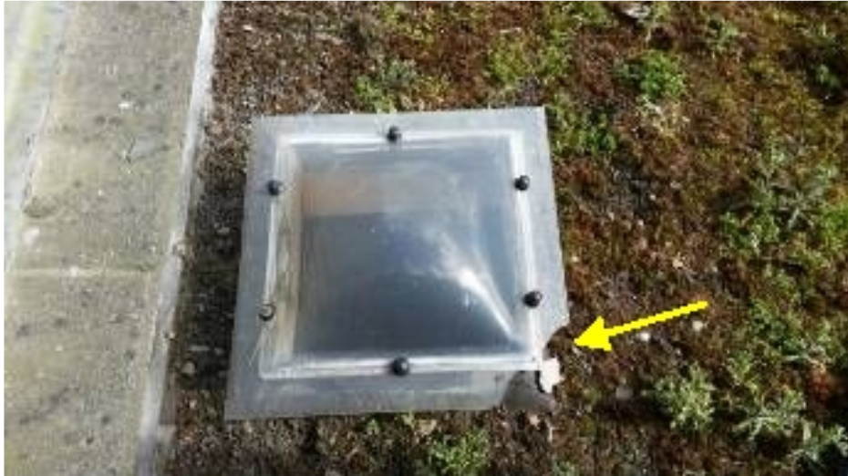
Damaged skylight.
