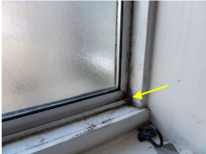
Mould around window frames.
