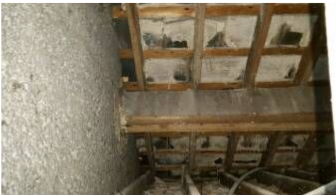
Main roof is constructed of traditional cut roof timbers.
