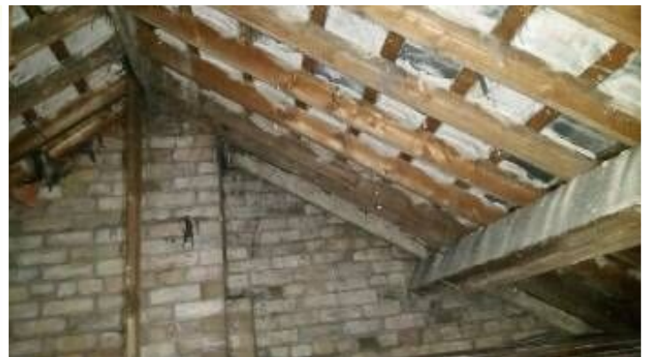
No collars fitted between roof rafters in roof structure, fit collars.
