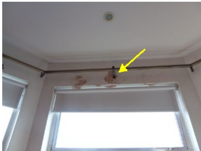
Moisture penetration through exterior wall.
