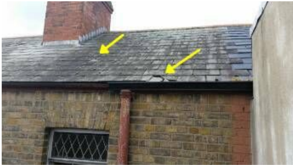
Slipped roof coverings.
