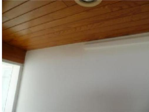
19. **Interior: Ventilation:** No vents opening fitted, ventilation through old windows not closing to frames, gaps.
