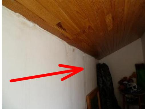
18. **Interior: Ceilings:** Timber panelled ceiling. Numerous old leaks from roof.
