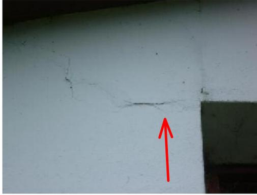
14. **Type of Structure to Extension.** Masonry structure Floor lifting in side sunroom extension, likely pyrite expansion.
